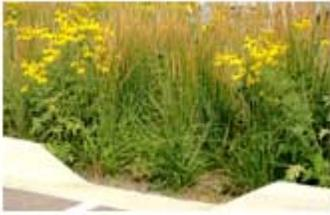
Another component of the parking lot are bioswales. Bioswales clean the water. Stormwater run-off that does not seep into the gravel is directed to a bioswale via cuts in the barrier curb. A bioswale is a slightly concave planted median between the parking areas. The surface is modestly sloped so the water moves down grade and passes through specially selected plants. The plants help remove particulates and pollutants from the running water.
