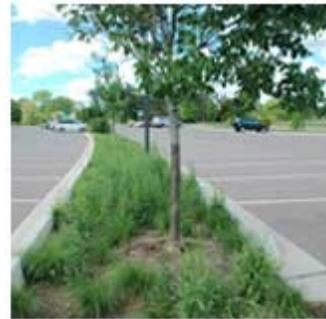
The water then flows out of the system into a created wetland, where it is further filtered before flowing into Meadow Lake and the DuPage River.
