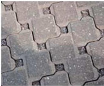
The Morton Arboretum's environmentally friendly main parking lot reduces pollution, erosion, and flooding because it absorbs stormwater rather than allowing it to run directly into storm drains, detention facilities or streams. Its design slows, cleans, and cools rainwater run-off before it enters Meadow Lake and the DuPage River.
